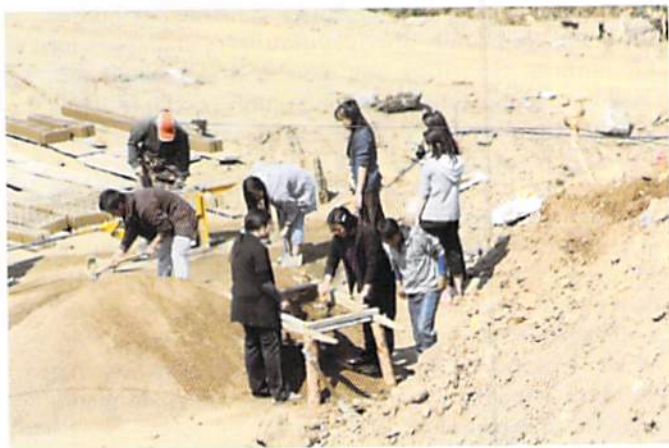
Students constructing house in Kanglung
